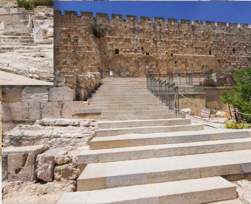
Small shops, which had a narrow street built above them, were built along the southern wall of the Temple Mount.
